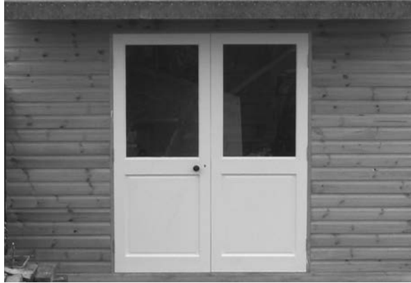
Front elevation, newly-constructed, 2005.
