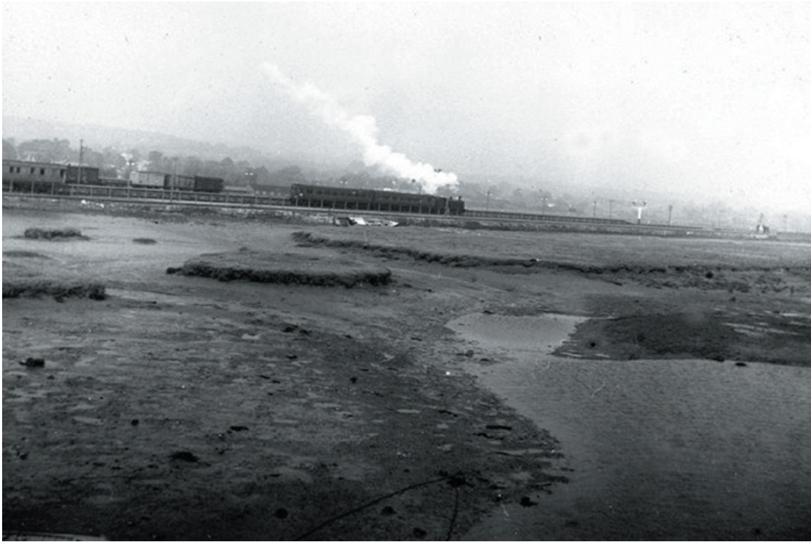
Axe branch embankment level line low marsh railway river salt signal steam tide valley
