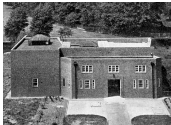
The acoustics building for testing and research at the National Physical Laboratory, Teddington, 1930s.
